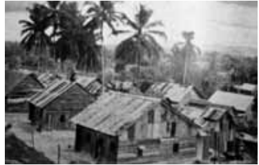
Chinese villages - built during the Emergency period
